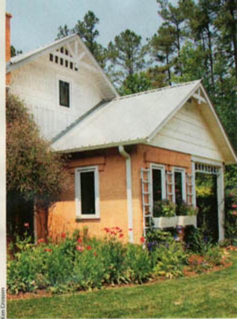
Galvanized steel roofs, either painted or unpainted, are affordable and durable, with a life expectancy of up to 100 years.
