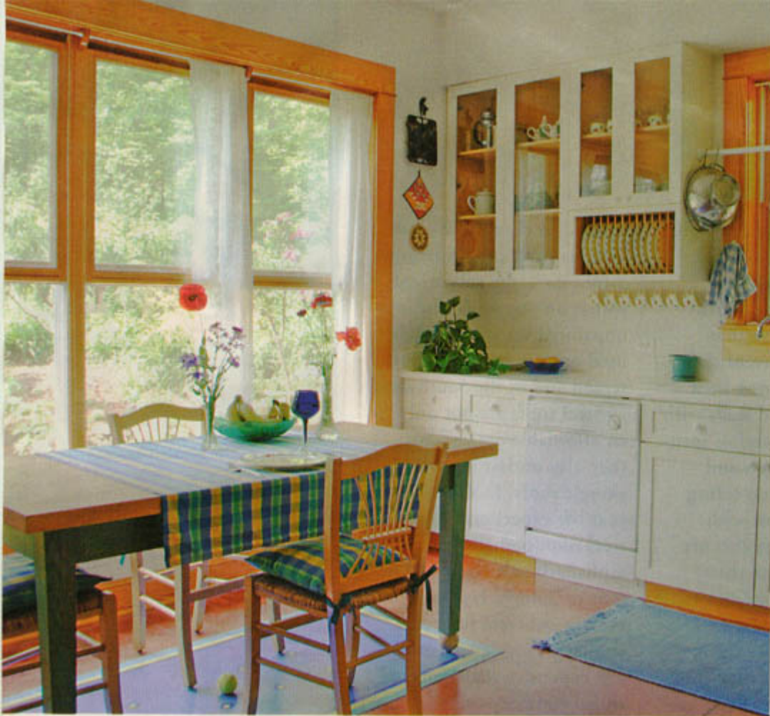
LEFT and BELOW: Four-inch-thick colored concrete flooring is warmed by a radiant hydronic heat system.
