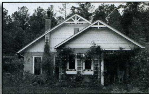
When leafed out during summertime, vines help shield these east-facing windows from the morning sun.
