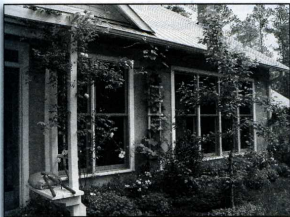
The wide overhang on the south side of Kathleen Jardine and Jim Cameron's home blocks the higher rays of the midday summer sun.
