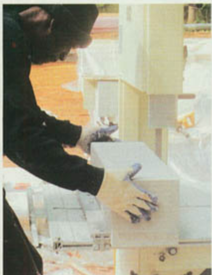
It's not wood but cuts like it. Hebel block can be cut with standard wood-working tools, such as a bandsaw. This saw was rented from Hebel.
